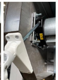
If a 45° box is not fitted, secure the knuckle to the endplate flange.
