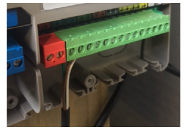
Pre-wired block in place
